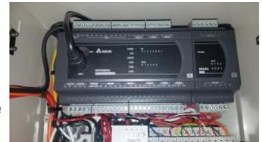
Section 3 Delta CPU and Output Module
