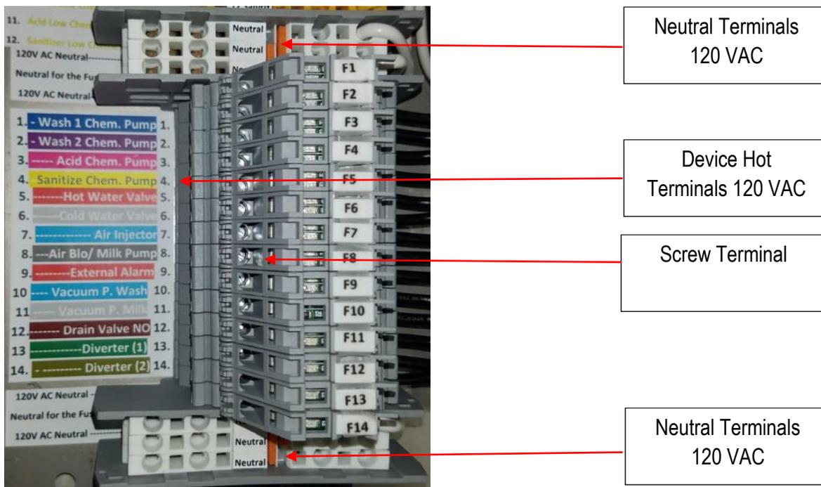
Loosen terminal contact with a flat blade screwdriver. Then insert wire for device and connect other wire to device to a neutral terminal. See Page 10 on how to connect to the neutral terminal.
