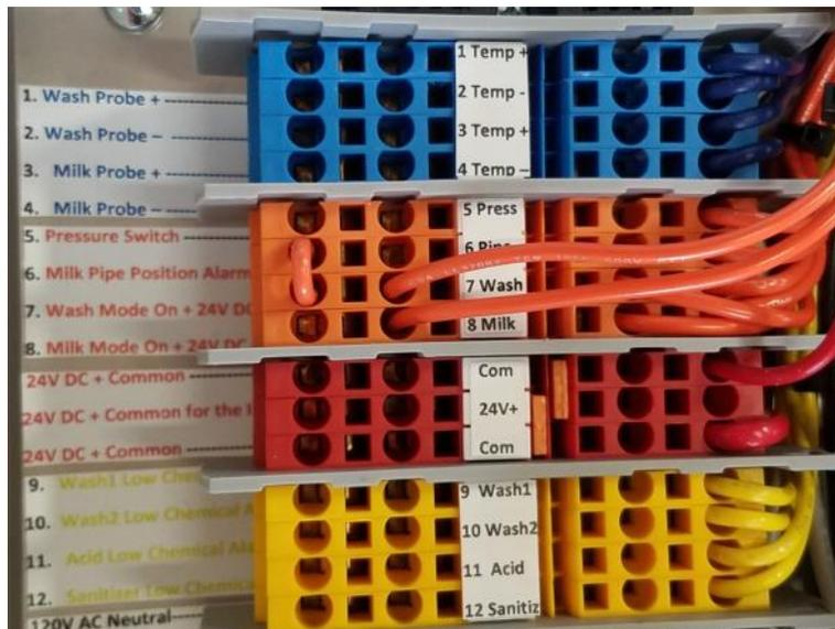
The orange and yellow inputs are looking for a connection from the 24(+)VDC red terminals to make the activation of the device.
