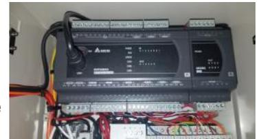
Section 3 Delta CPU and Output Module
