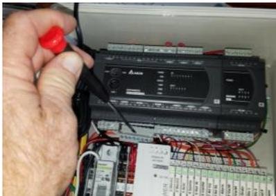
The CPU / Output Module can be removed from the din rail by releasing the 3 white tabs on the bottom side of the modules.
