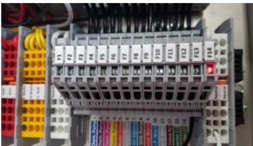
Now on the device output in question, press and hold that **OUTPUT** button to see if the fuse holder's red LED lights up.
