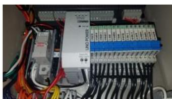
For the Inputs, test that they are wired correctly by activating them with the Test Kit Switches and Jumpers you hooked up earlier.
